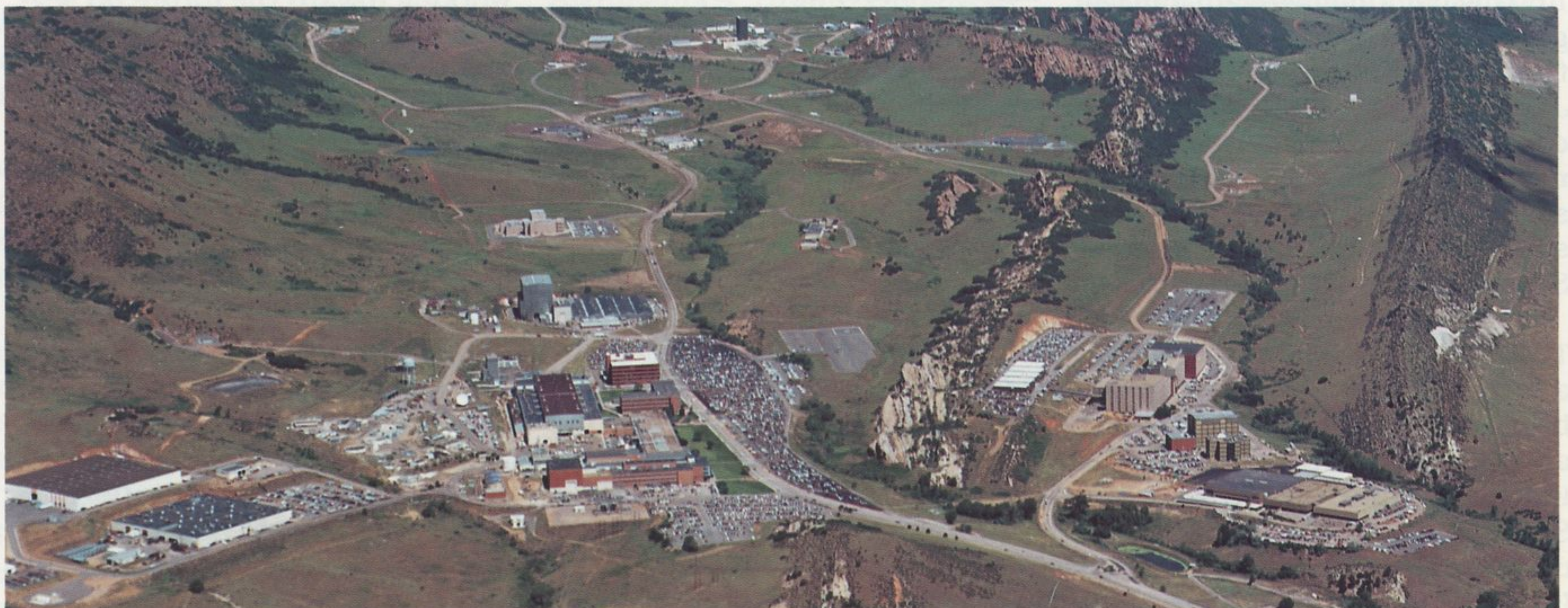
Main plant at Waterton
