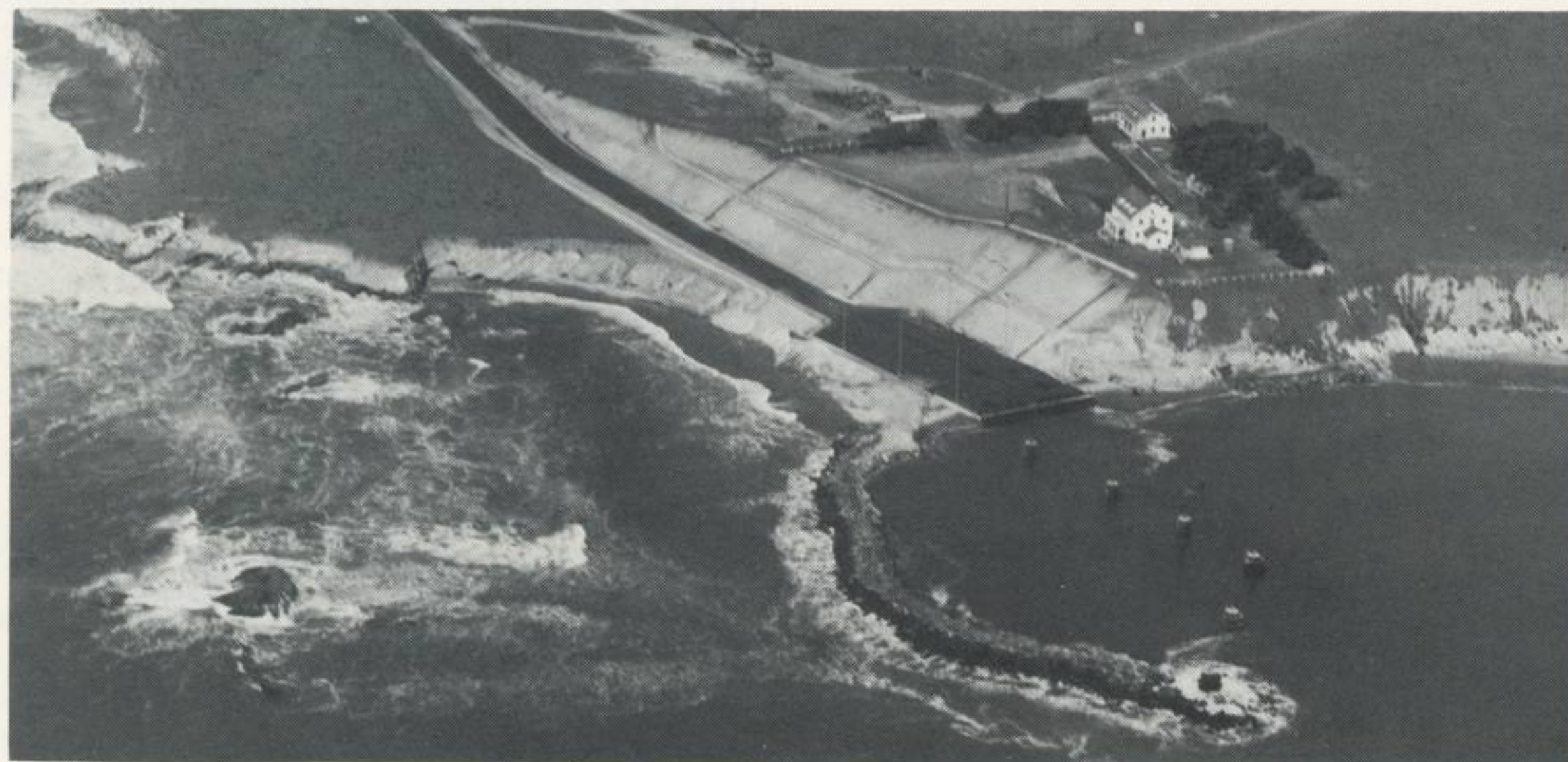
California harbor for external tank.
