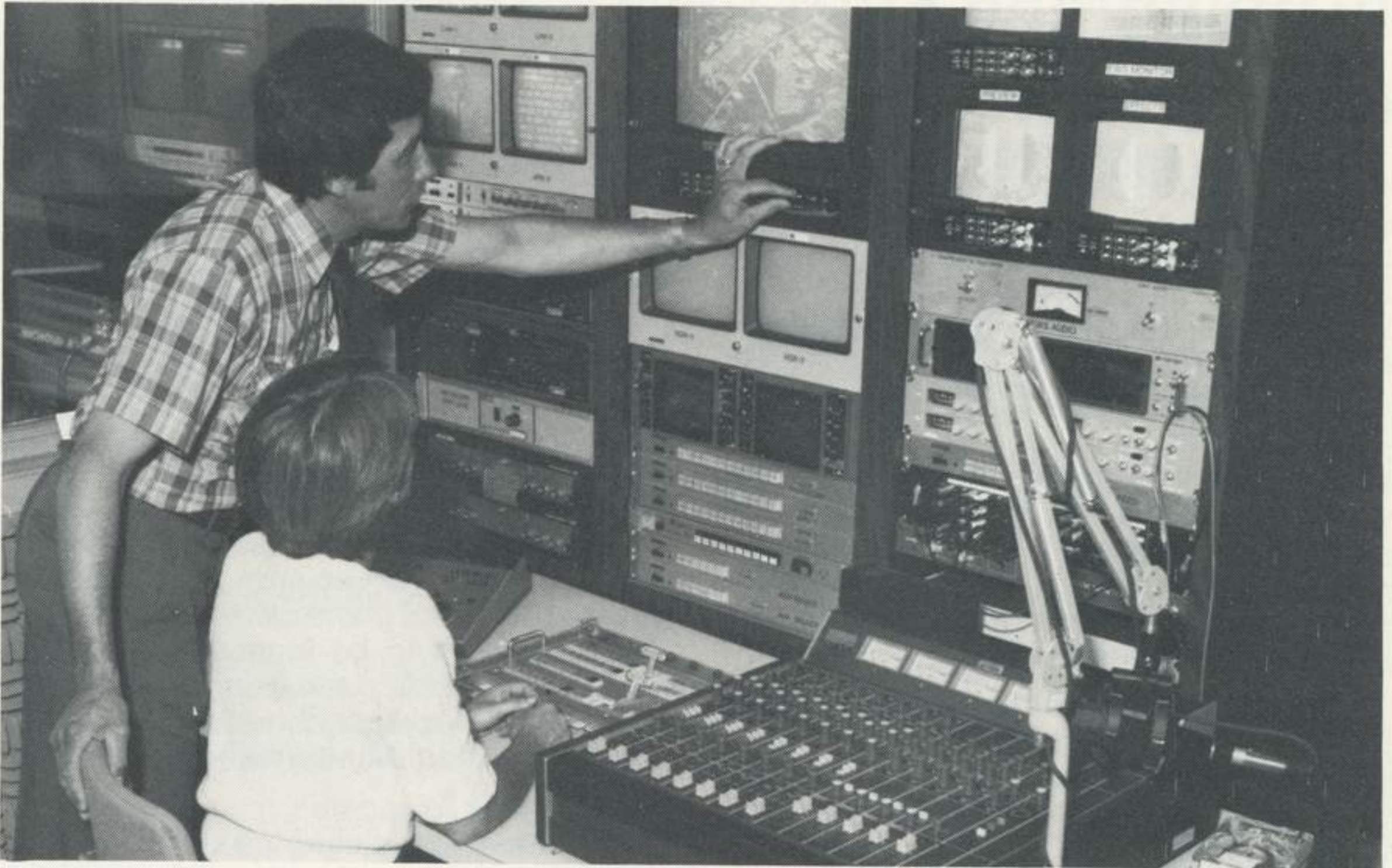
A new closed-circuit television system — the emergency warning system (EWS) — has been installed at Denver Aerospace's Michoud division, New Orleans to warn personnel of emergencies and alert them to general information. Seventy television monitors throughout the facility give off an audio signal, followed by a voice announcement. The EWS studio has the capabilities of a complete video and audio closed-circuit television station, using a microwave broadcast system. Addition of a satellite receiver dish soon will enable Michoud to pickup NASA feeds, transmitted directly during space shuttle missions, as well as national weather advisories. Jay Heitzman (left), senior video operator, and Lisa MacDowell, audio/visual technician, are shown checking an on-air monitor at the EWS console.
