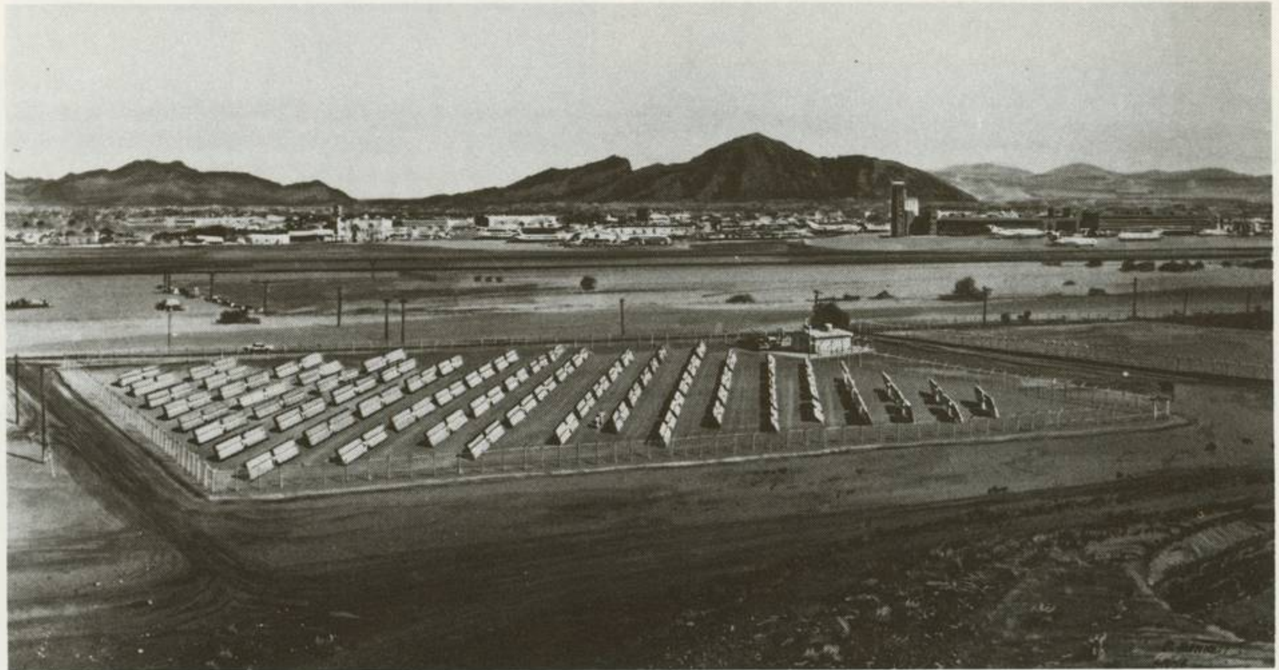
The solar photovoltaic power plant at Sky Harbor International Airport near Phoenix produces 225 kilowatts using 80 solar arrays, compared with 350 kilowatts from 160 arrays at the Saudi solar plant. Both systems were designed and built here.
