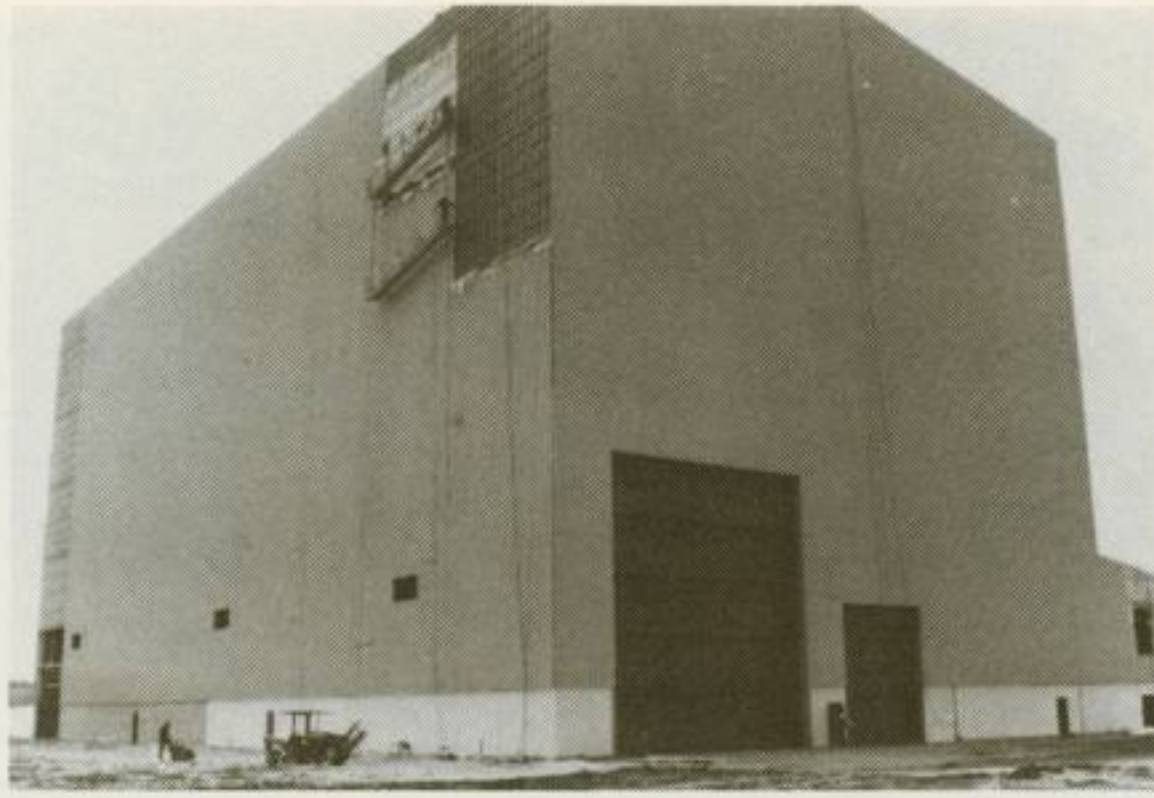
The top photos show the outside and inside of the missile assembly building under construction at Vandenberg Air Force Base. At right is the integration test facility for the MX.
