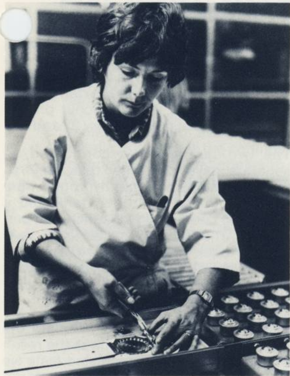
Rose Fitzmaurice connects a photovoltaic cell to a bypass diode on the photovoltaic assembly line. The cell and diode are mounted on an aluminum heat diffuser.
