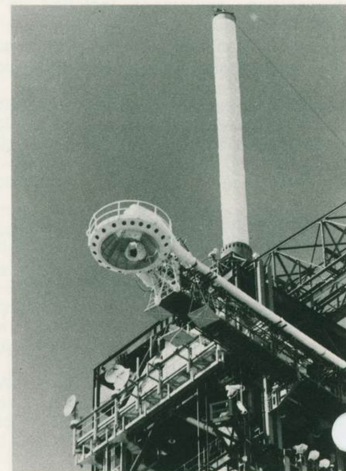
The gaseous oxygen vent hood, center, seals over the external tank nose cone to prevent ice formation. The tall structure is an 80-ft-high, 5-ft-dia lightning rod.
