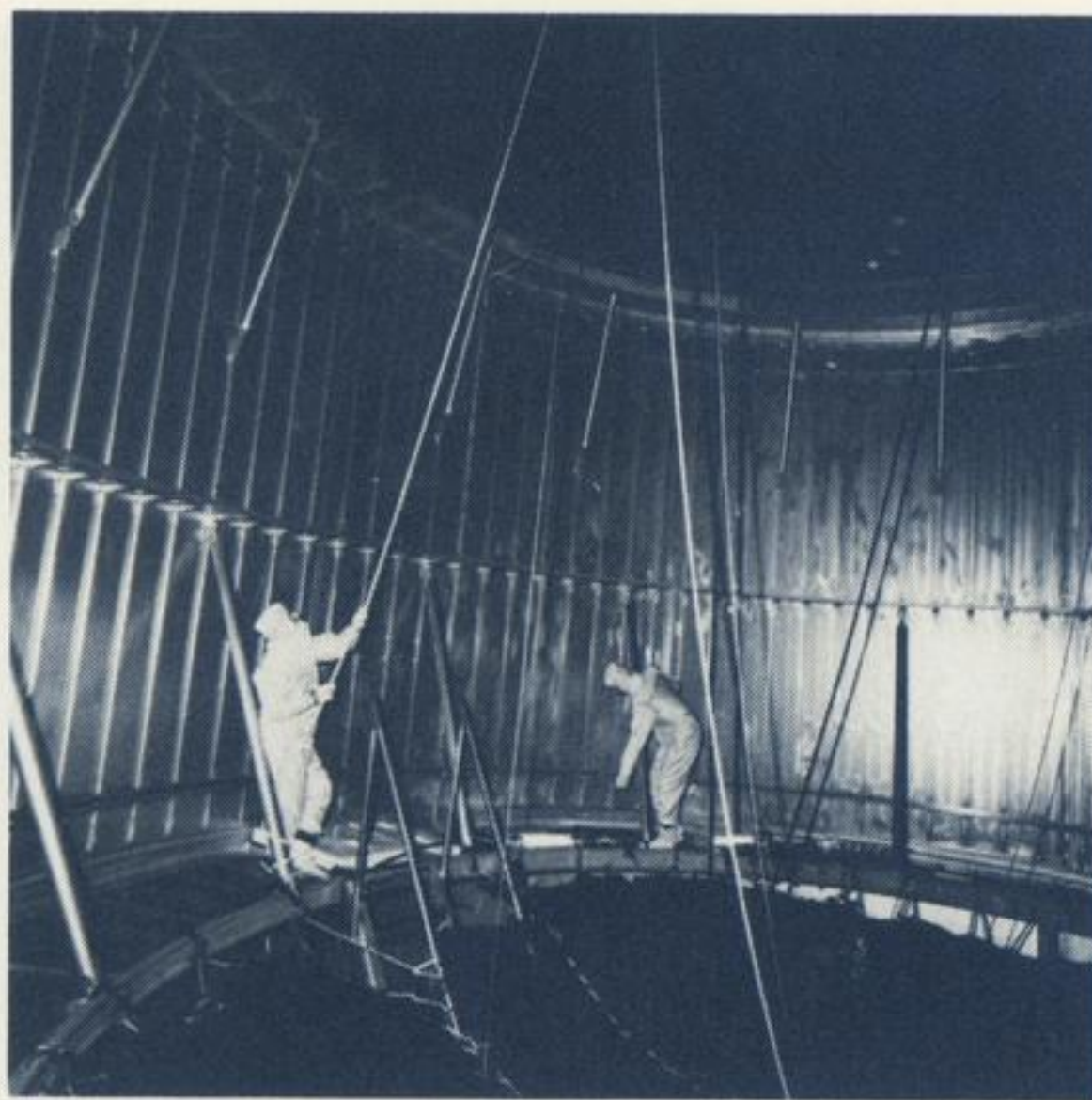
External tank operations employees work on modifications inside the liquid hydrogen tank at Kennedy Space Center. In the first photo, one of two tripod assemblies that help stabilize the two-person movable platform during assembly and dismantling is installed. Tag lines leading to a swiveling beam assembly are checked in the center photo. In the photo at right, the platform is raised inside the 97-foot long liquid hydrogen tank. The platform, attached to a swiveling beam assembly, can rotate 360 degrees to permit access to the total length of the tank.
