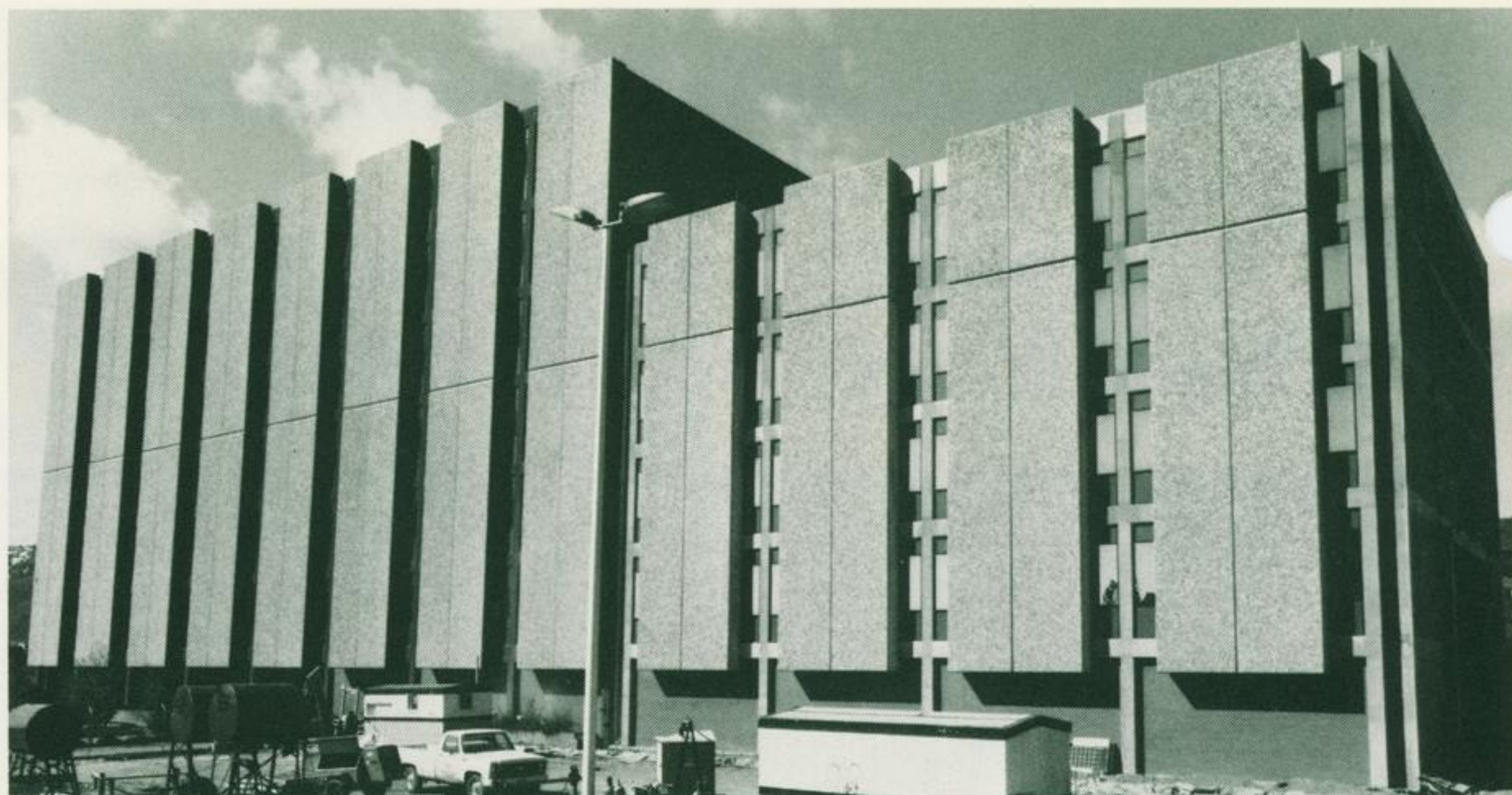
Near-field antenna test facility was added, at right, to SSB.
