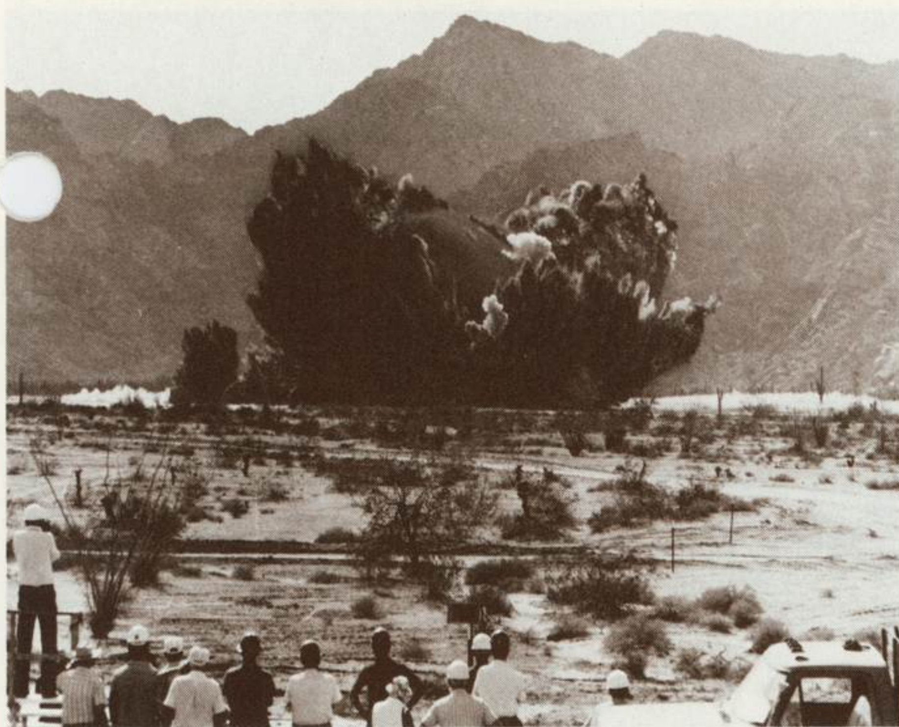
Some 13,600 pounds of high explosives are detonated at left to test the design of an underground blast protective device for the proposed Missile X system. The device, called a blast plug, is shown at right after the test. In the Arizona desert near Yuma, the Air Force conducted the test on the blast plug developed by the Denver Division. The test simulated the effects of a nuclear blast on the 64-foot long, 296,000-pound steel plug placed in an underground reinforced concrete tunnel. The tunnel is one of several multiple aiming point basing concepts being studied for the proposed Missile X intercontinental ballistic missile.
