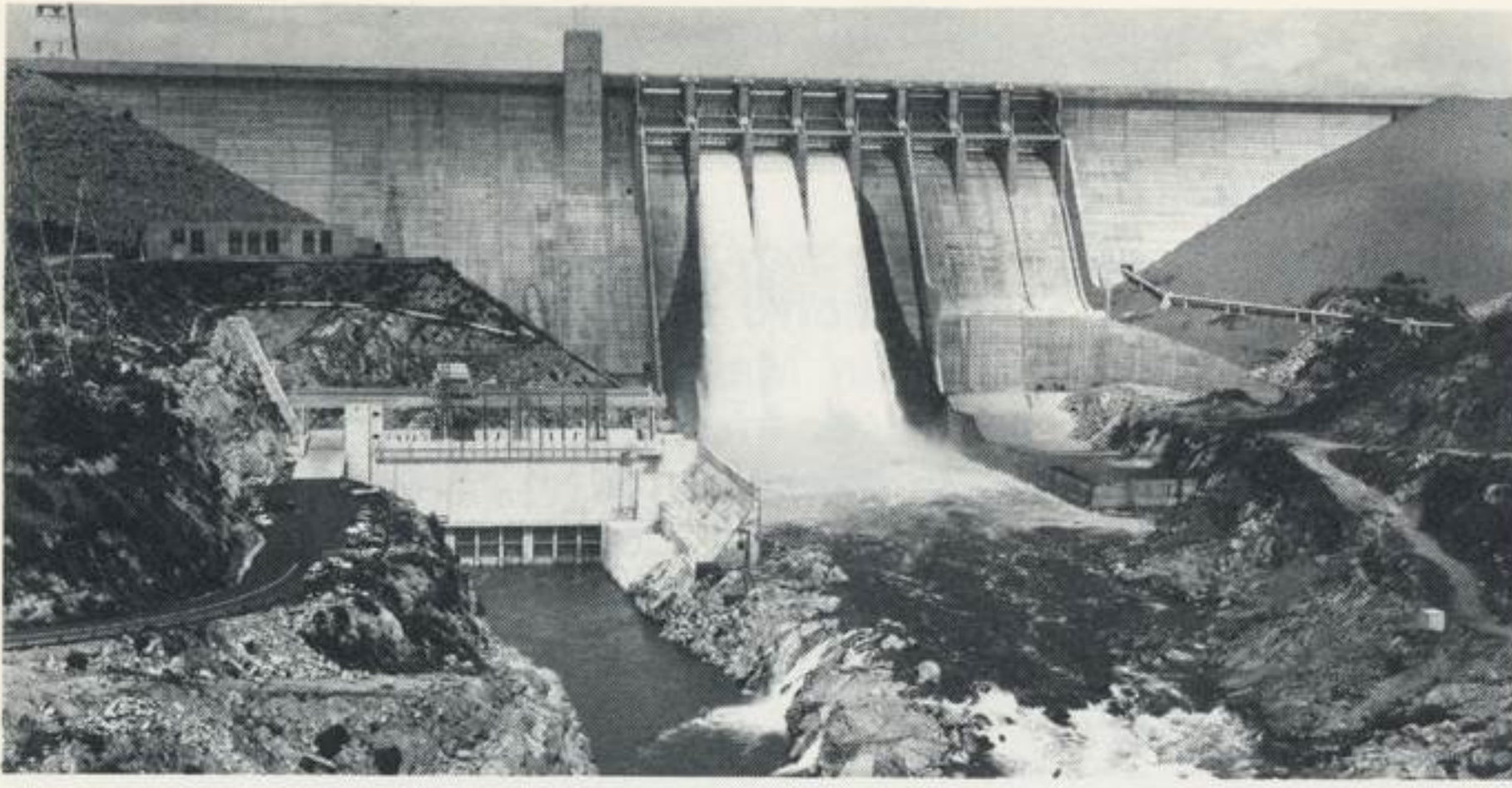
Folsom Dam and power plant are in operation.
