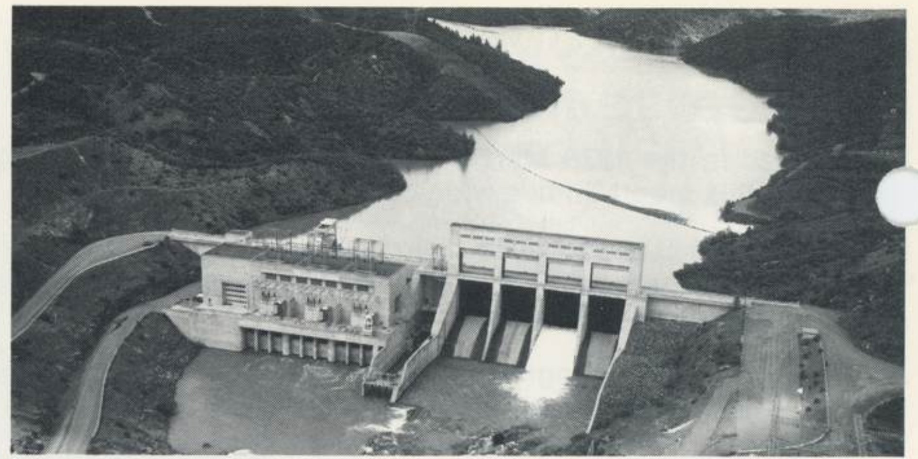
Keswick Dam equipment is being installed.
