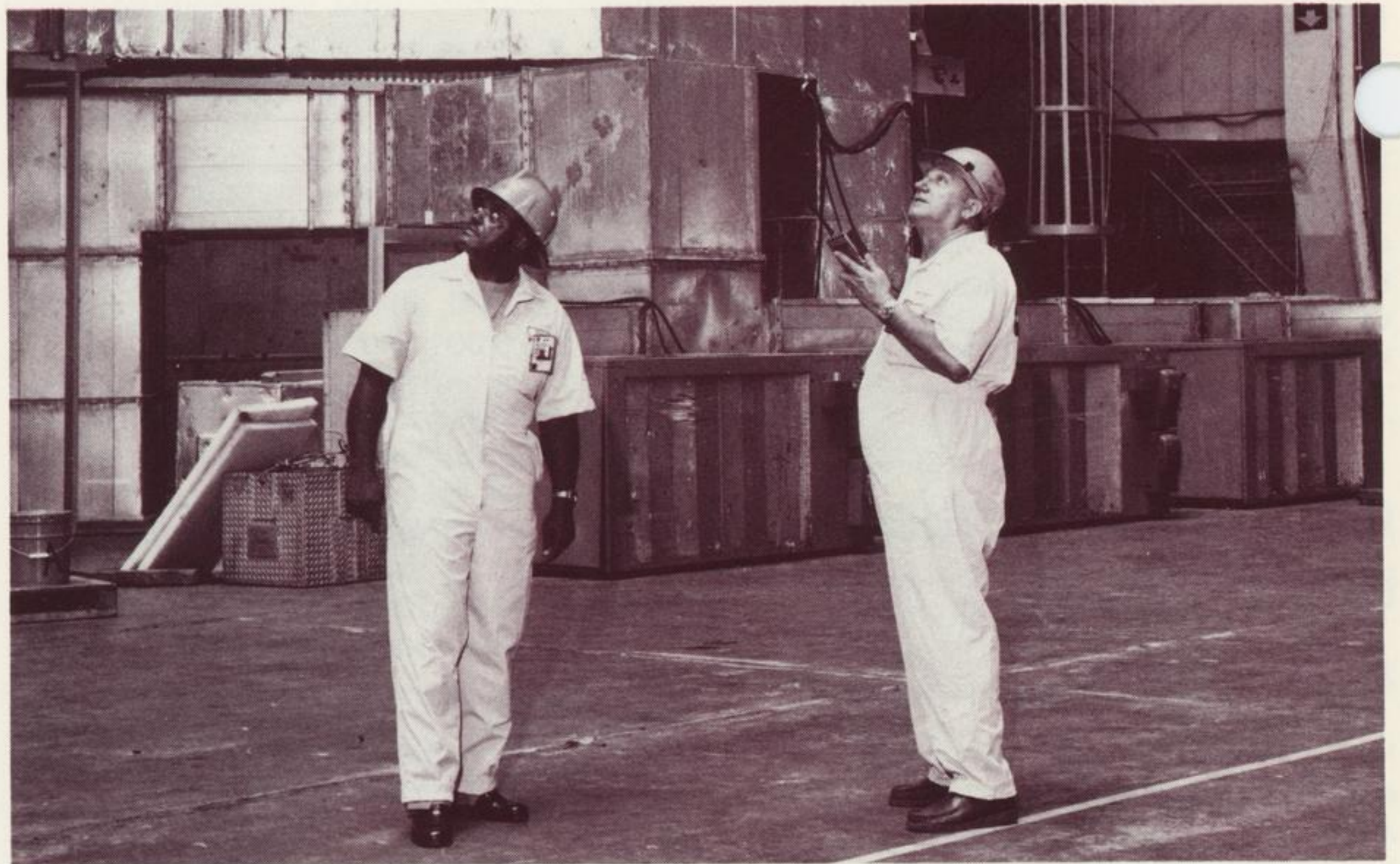
Floor talker Leo Veron, right, gives radio instructions to Mitchell McAlister who is more than 200 feet above him in the overhead crane cab. At left is Herman Jolly, who supervised the move of the liquid hydrogen tank from cell B to cell C.
