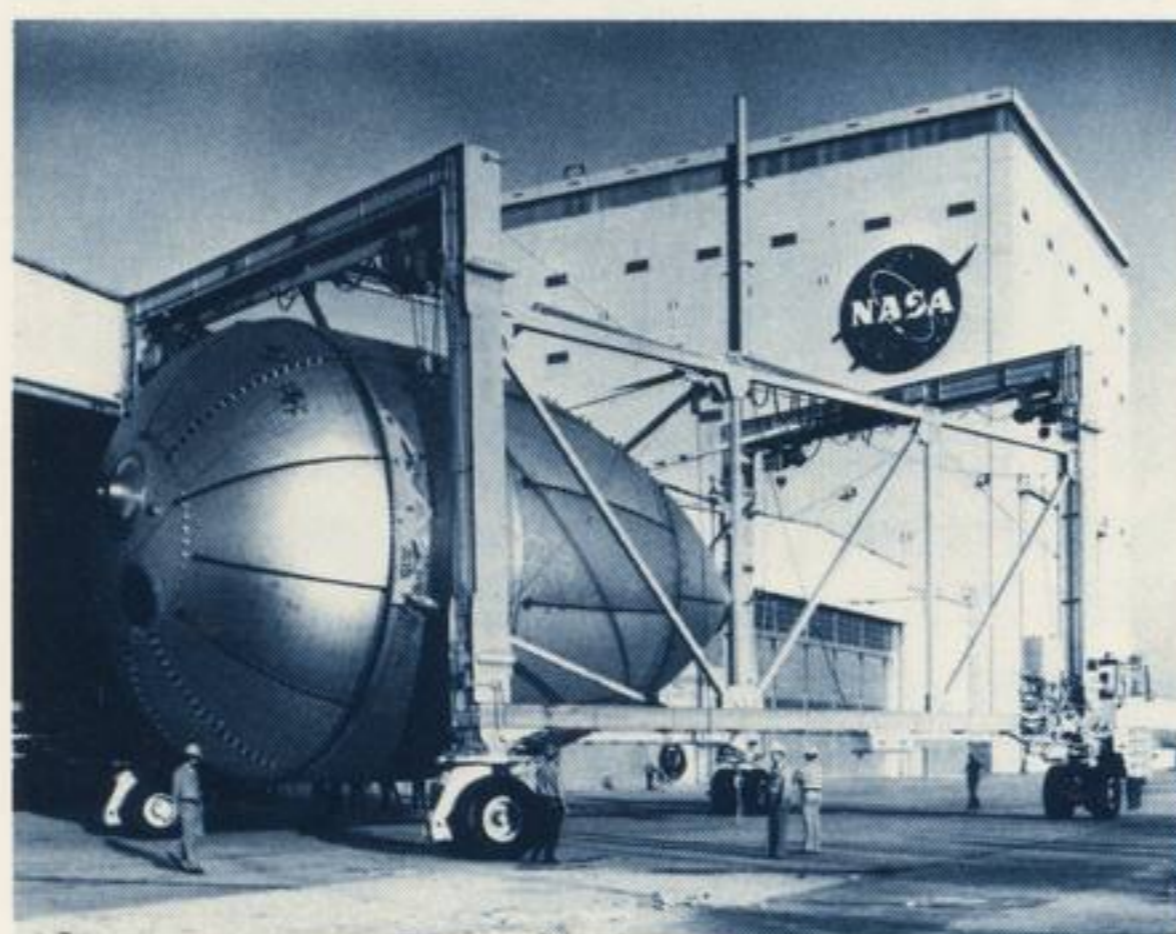
Liquid oxygen tank is moved by straddle to the vehicle assembly building (top) and then lifted into the hydrostatic test cell (bottom).
