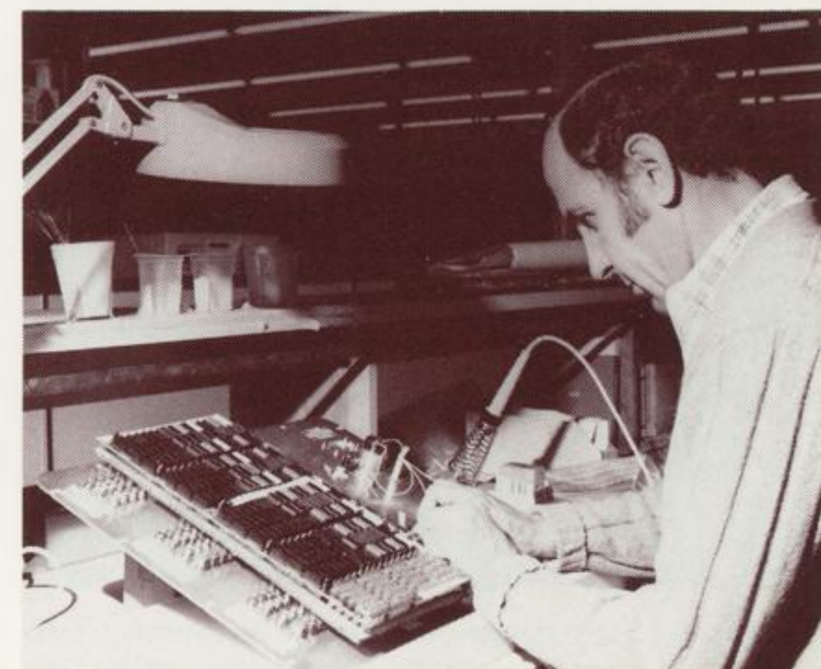
Morse Galitello assembles a wire wrap board, one of the components of the CCMS.
