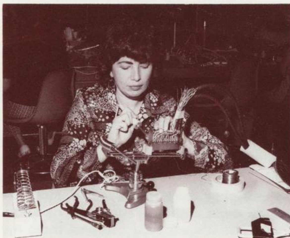
L. M. Collier completes a terminal on analyzer cable.
