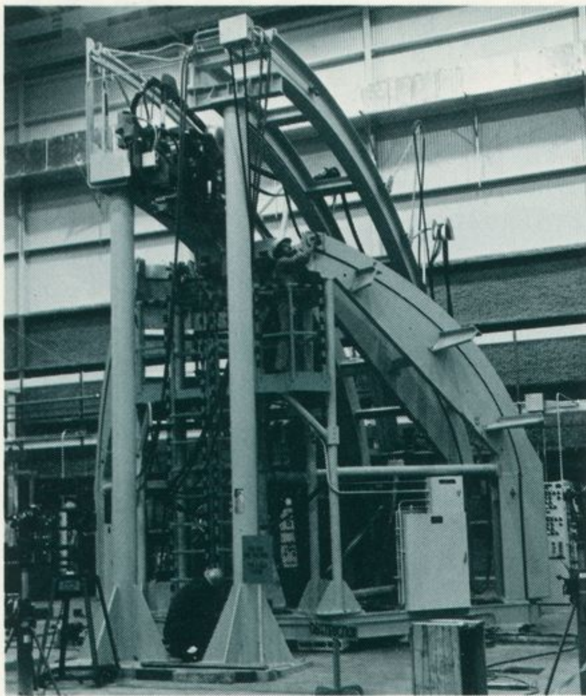
First formal use of the dome gore trim and weld tool shown here was made in September at the Michoud Operations in New Orleans when first Space Shuttle external tank production-type welds were completed. Results of x-ray and visual checks showed welds to be excellent. The fixture is used to weld three gore panels into a one-quarter dome shape. Production could reach 180 domes each year, with the program anticipated to run until 1991.
