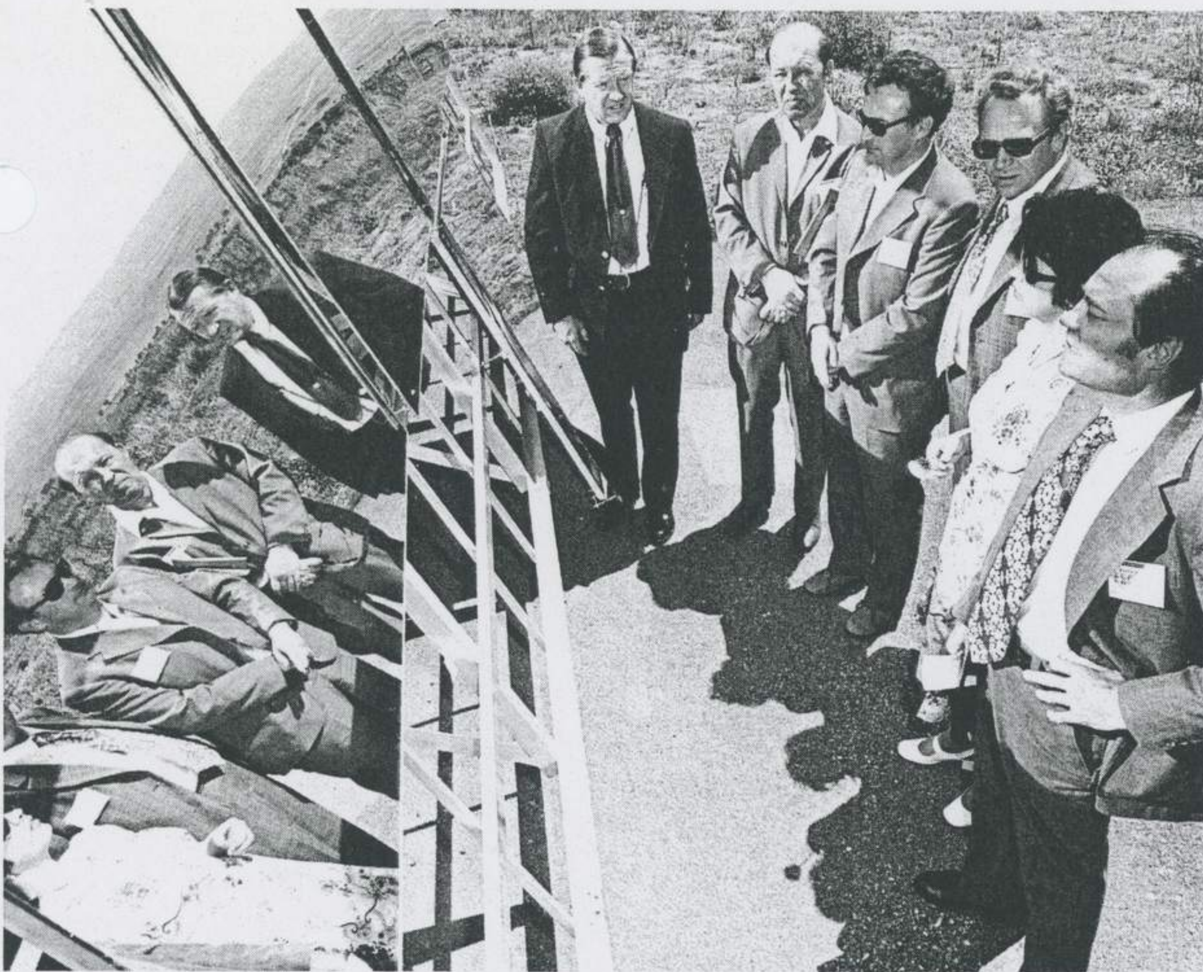
SOLAR ENERGY RESEARCH MIRRORS reflect the images of Soviet Union scientists visiting Martin Marietta Aerospace in Denver to review research currently underway to develop solar energy for heating and cooling buildings. These large, curved, concentrating heliostatic mirrors are the fundamental building blocks of
