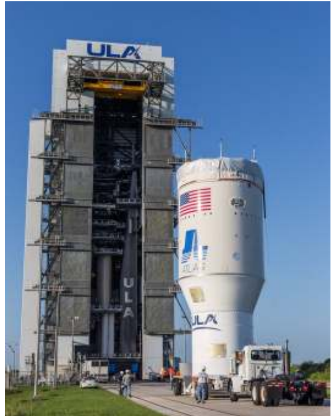
The Centaur upper stage, interstage adapter and the lower half of the Atlas 5's payload fairing were installed as a single unit on top of the launch vehicle June 10. Credit: United Launch Alliance
