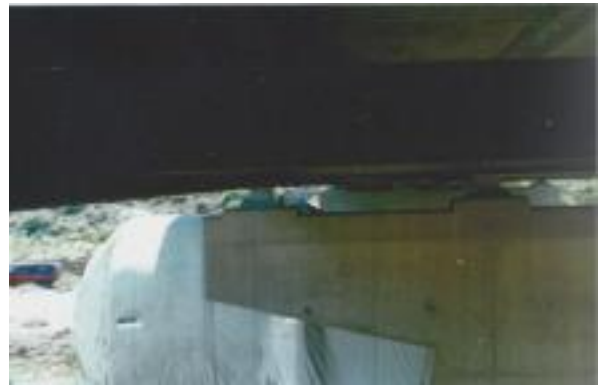
Photo # 3 Under the bridge
